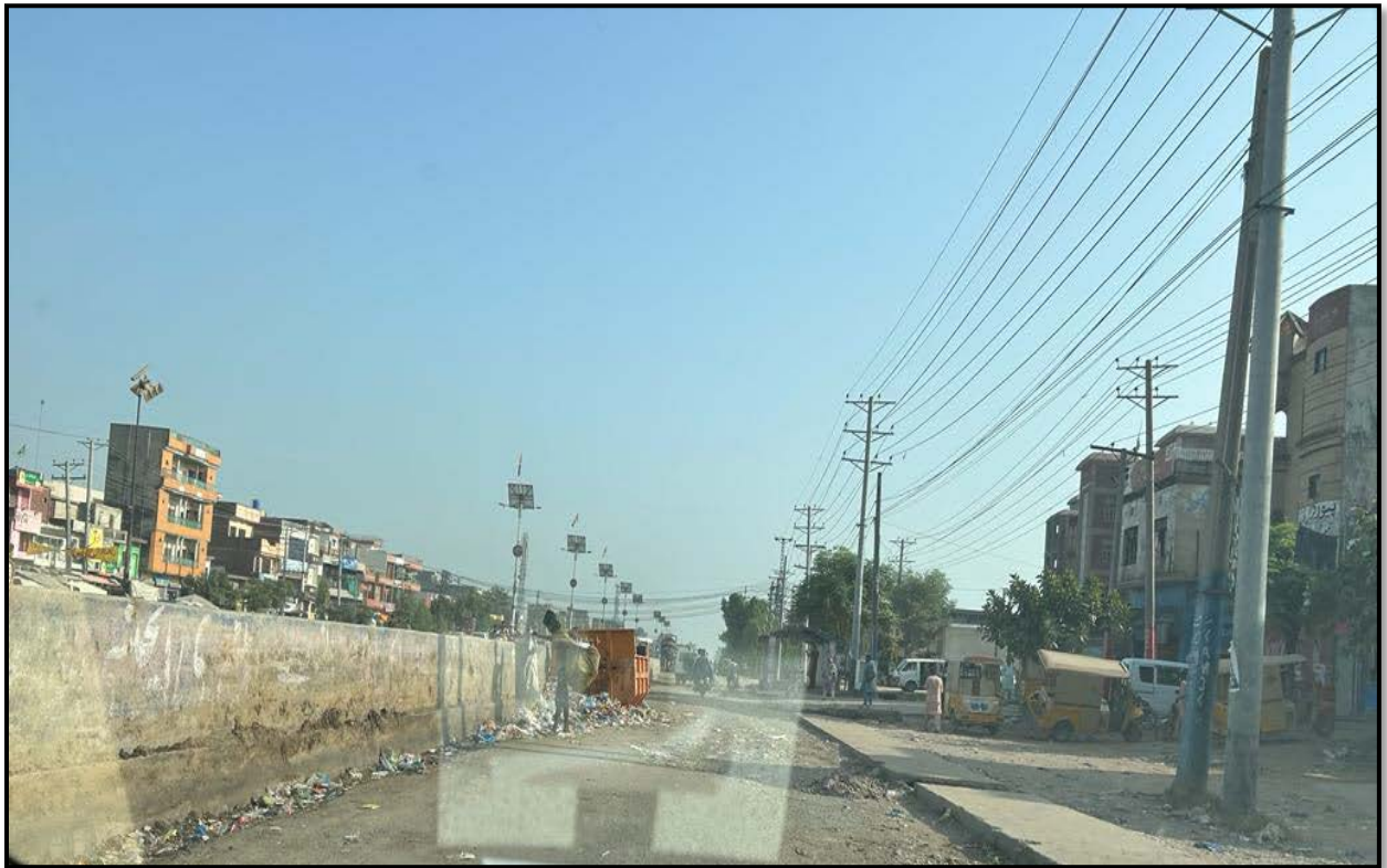
Fig. 1.2: A view of Drain along Service Road
