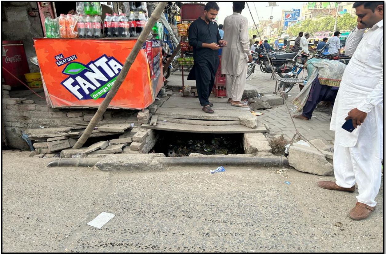
Fig. 1.1: A view of Drain along GT Road close to property line
