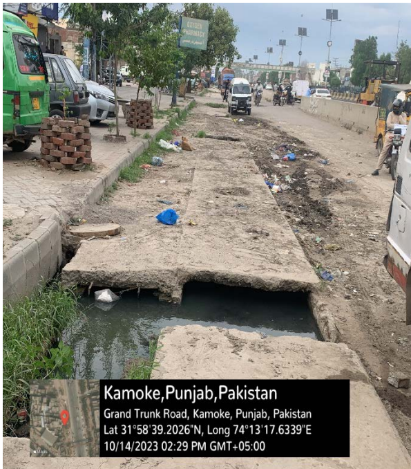
Existing drain without cover and ponding area on the road
