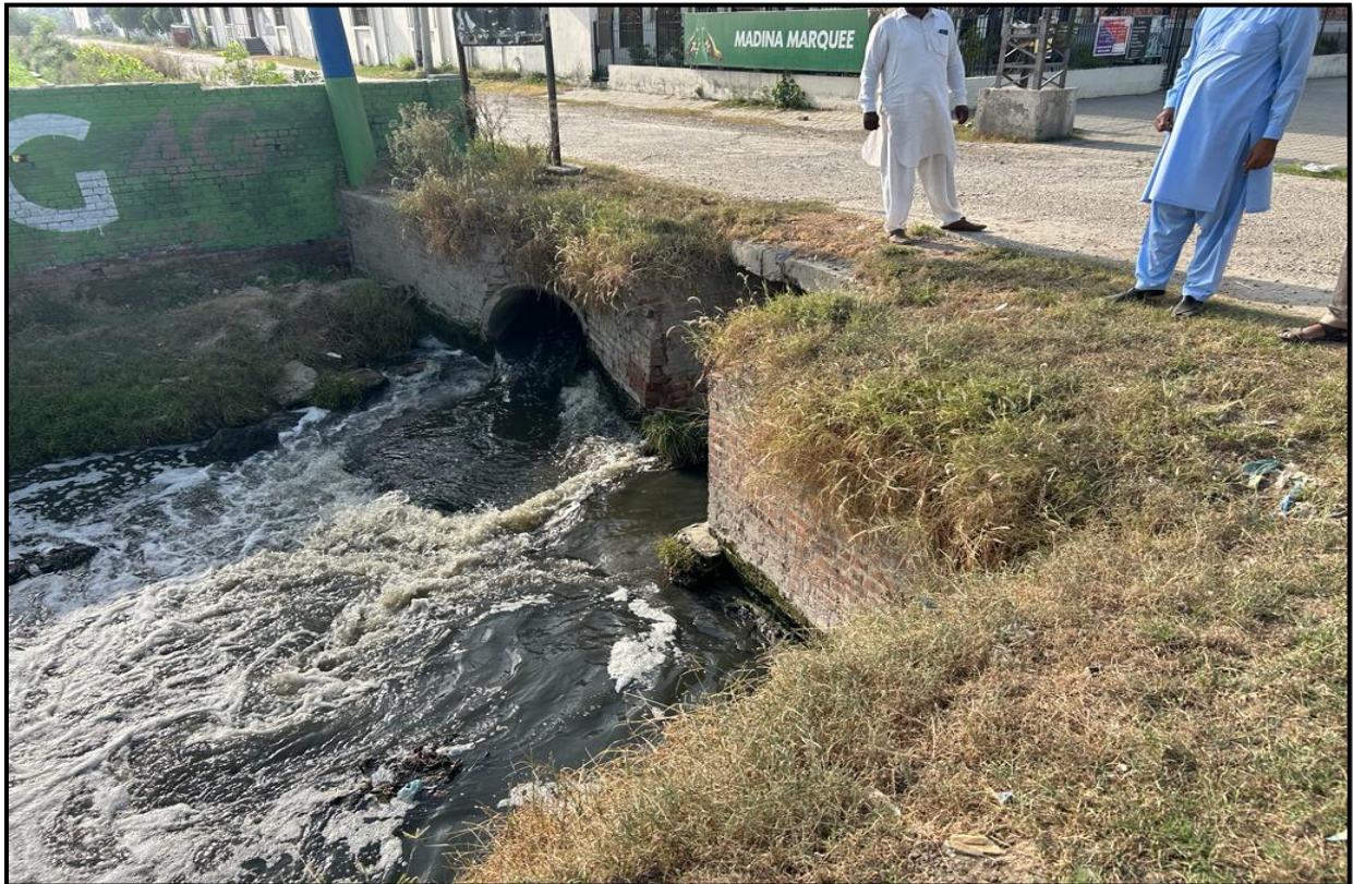
Fig. 1.4: A view of drains at outfall
