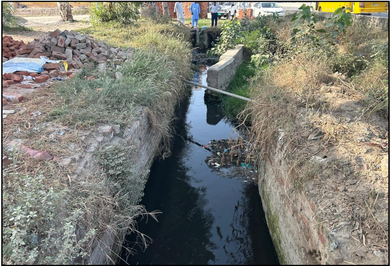
Fig. 1.3: A view of Drains falling into Ghania Drain
